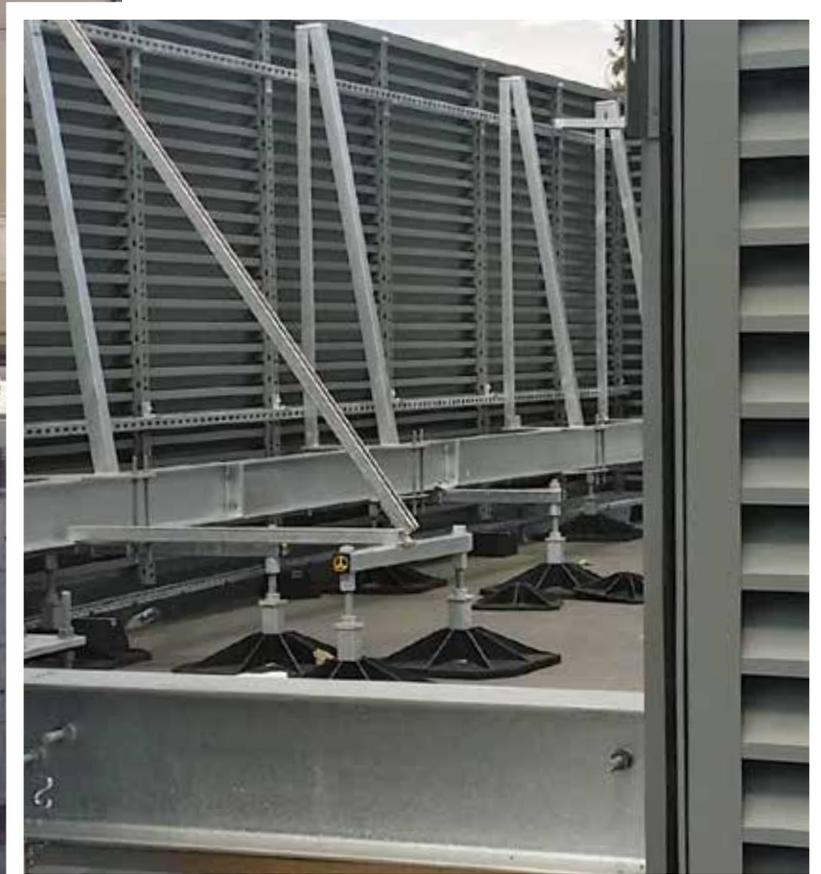
The adjustability of our system means that obstructions on the roof (sometimes not foreseen) can often be overcome without any significant modification
