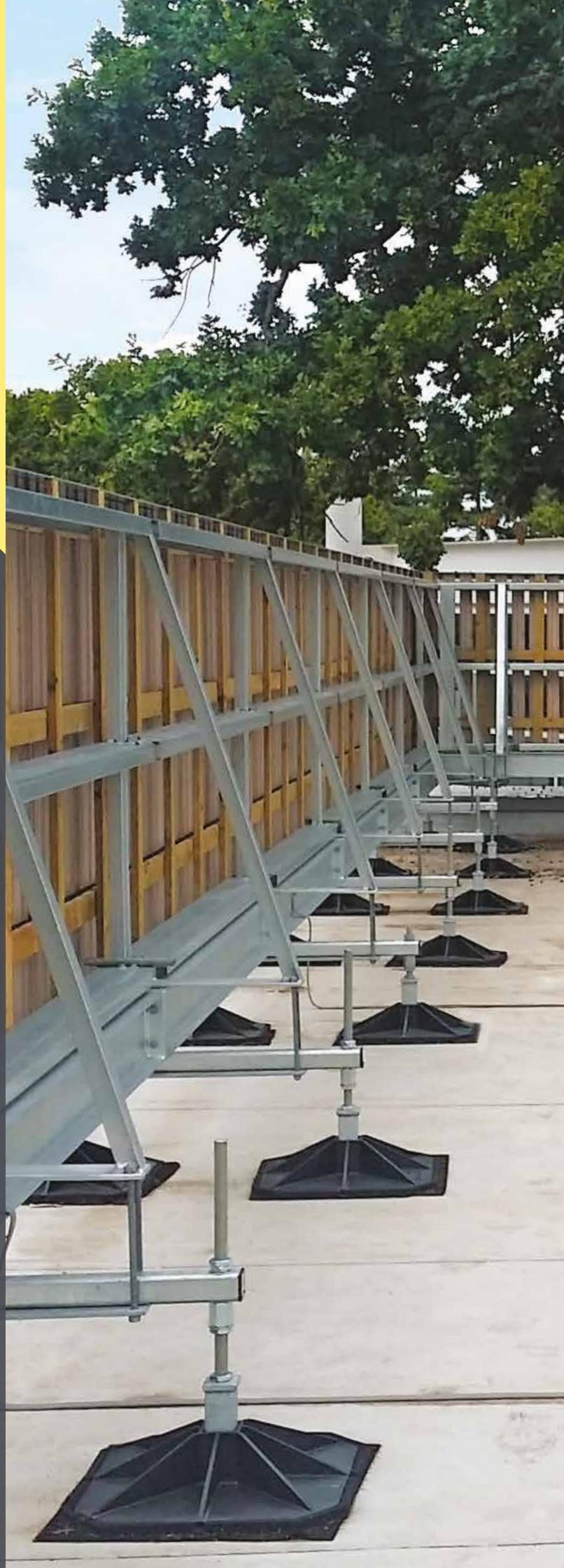
Big Foot Louvre Support Systems enable a non-penetrative installation that's quick and easy to install - designed specifically for the project
